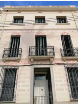
Vista façana principal
