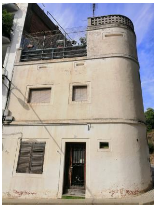
Vista façana principal
