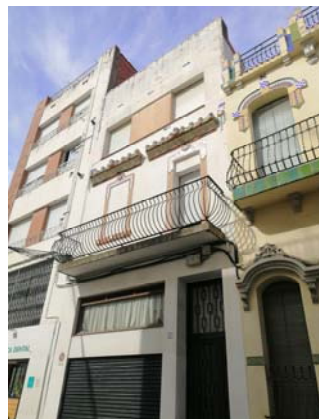
Vista façana principal
