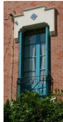
Detall obertura central façana principal
