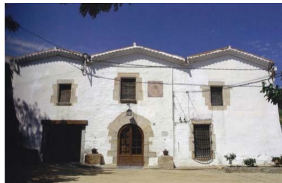
Vista façana principal
