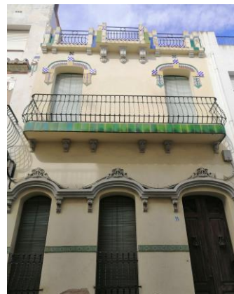
Vista façana principal
