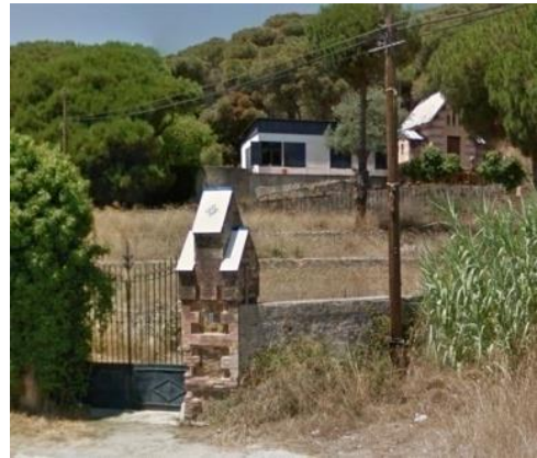
Vista façana principal
