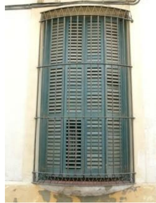
Detall obertura principal
