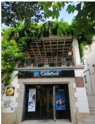
Vista façana principal
